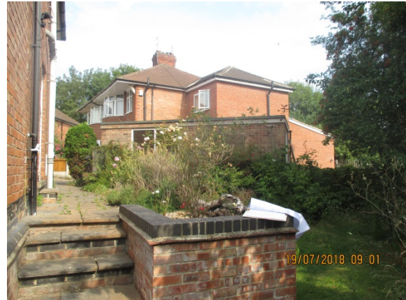
View of no. 57 from rear garden of site
